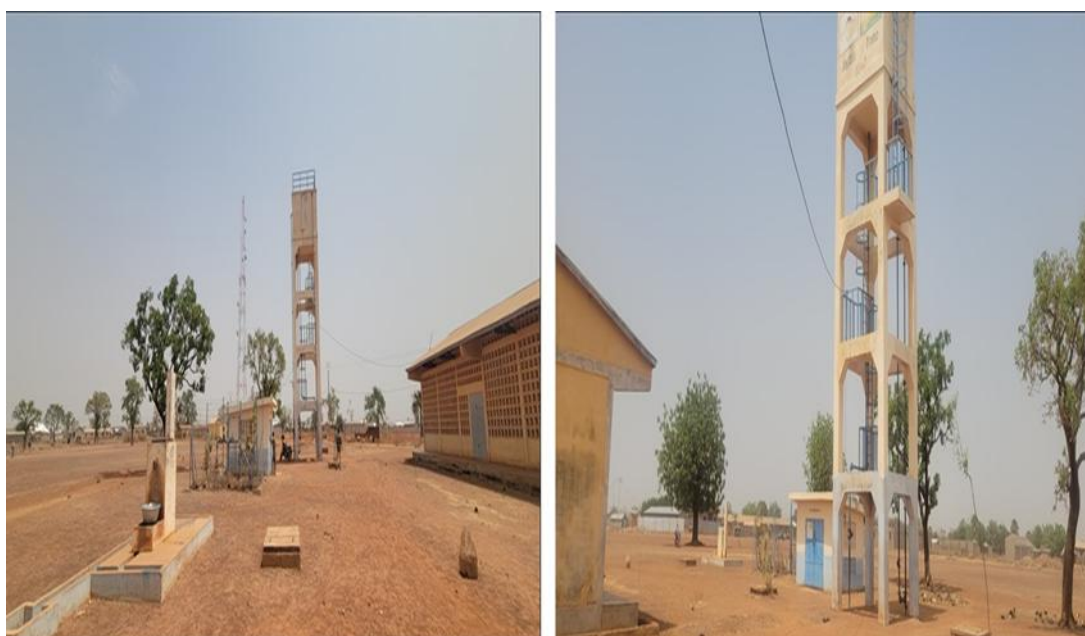
• b) The water tower to be rehabilitated, the catchment point and the technical room housing the genera
