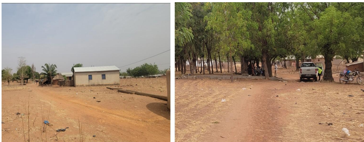
: Condition of the access roads intended for the passage of High Density Polyethylene (HDPE) pipes
