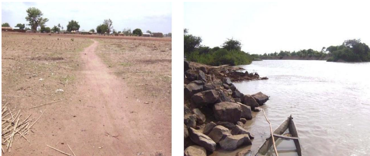
Condition of the tracks will serve as a passage for water supply lines and the appearance of the pumping point on the Kpendjal River Shot: Consultant, Bagré, February 2025.
